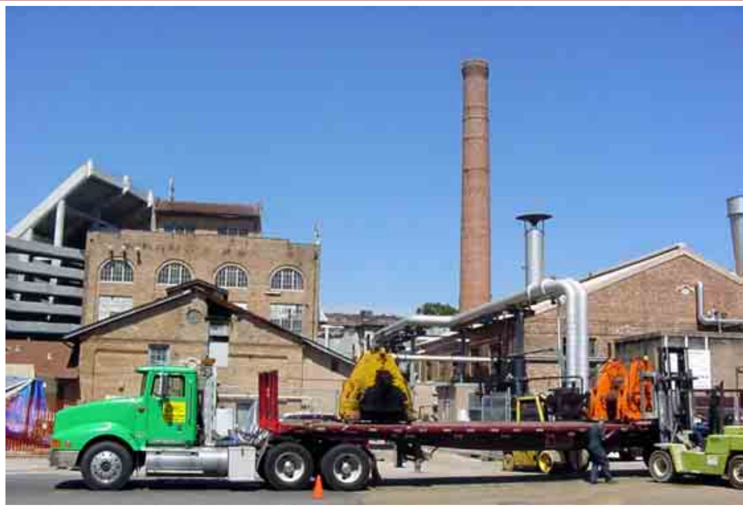
The 3-roll mills, the last remaining equipment from the Audubon Sugar Factory on the Baton Rouge campus, being removed for transport to St. Gabriel.
